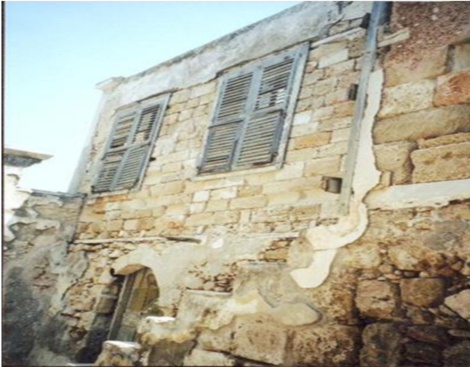
Picture 11- Present-day View of Rhodes Muftiate Office Building - 2014
