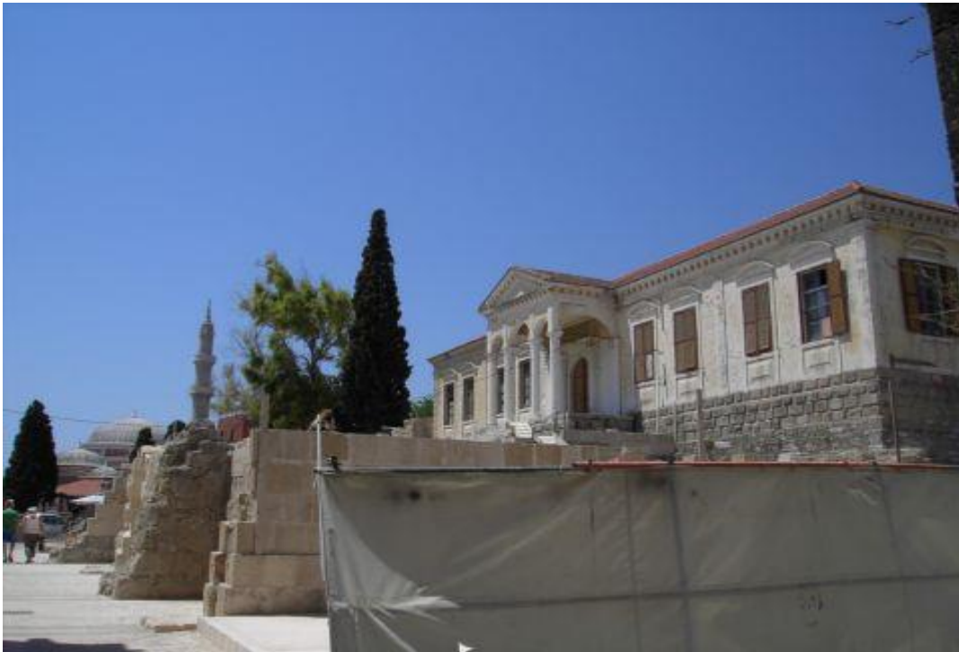
Ground Work Excavation at Suleymaniye Madrasah (2014)
